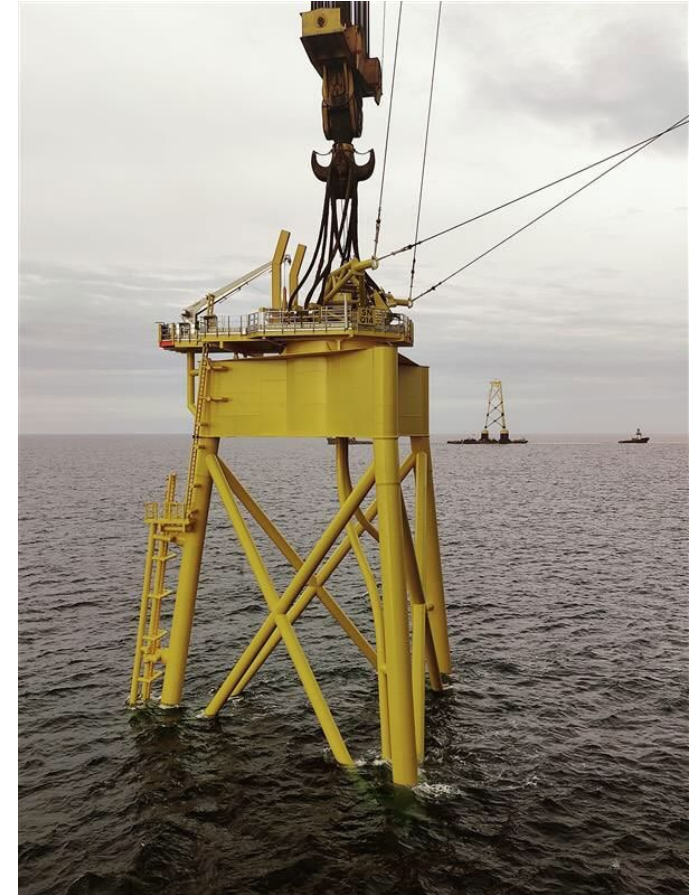
First jacket installed on the Seagreen project
